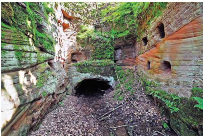
View east of the western portal of Eardington canal tunnel. Note the various holes and recesses in the cutting walls
